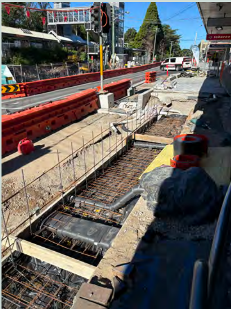
Pictured above; Hampden Road - work in progress!
