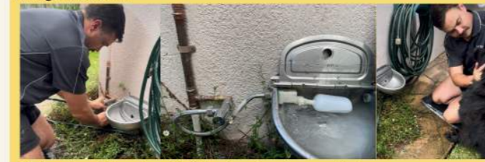
Rohan installing the self-filling bowl to the outside hose tap
